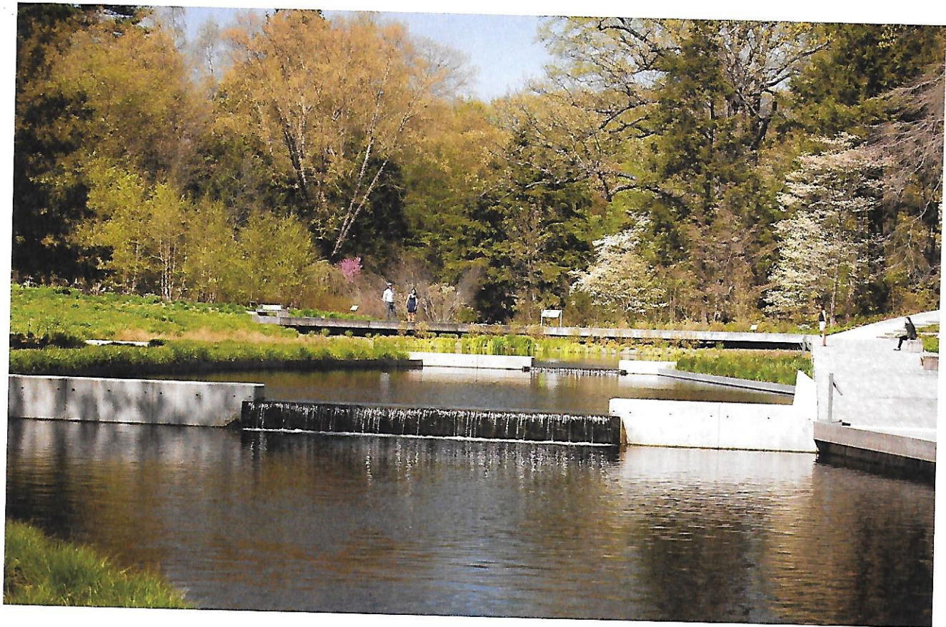
RIGHT Water flows down over two stone weirs, then back up through a massive underground cleansing system.
